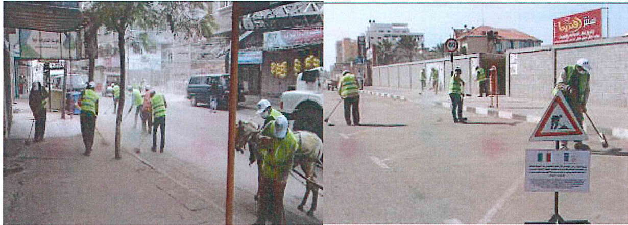
Construction debris & sand cleaning activity
