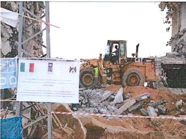
Rubble Removal Activities
