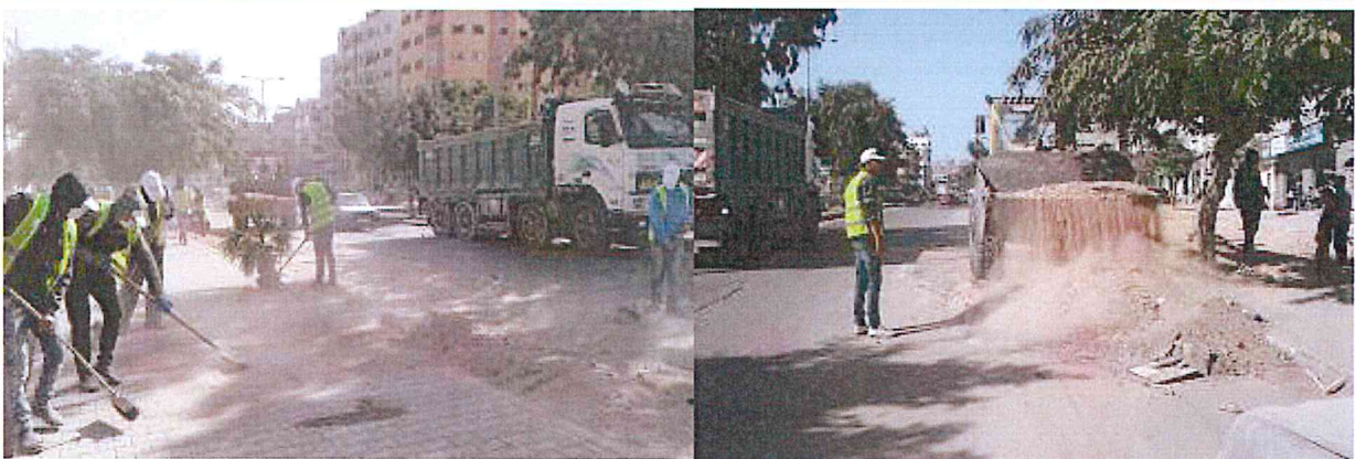
Construction debris & sand cleaning activity
