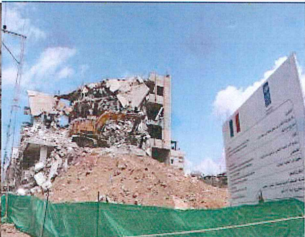
Rubble Removal Activities
