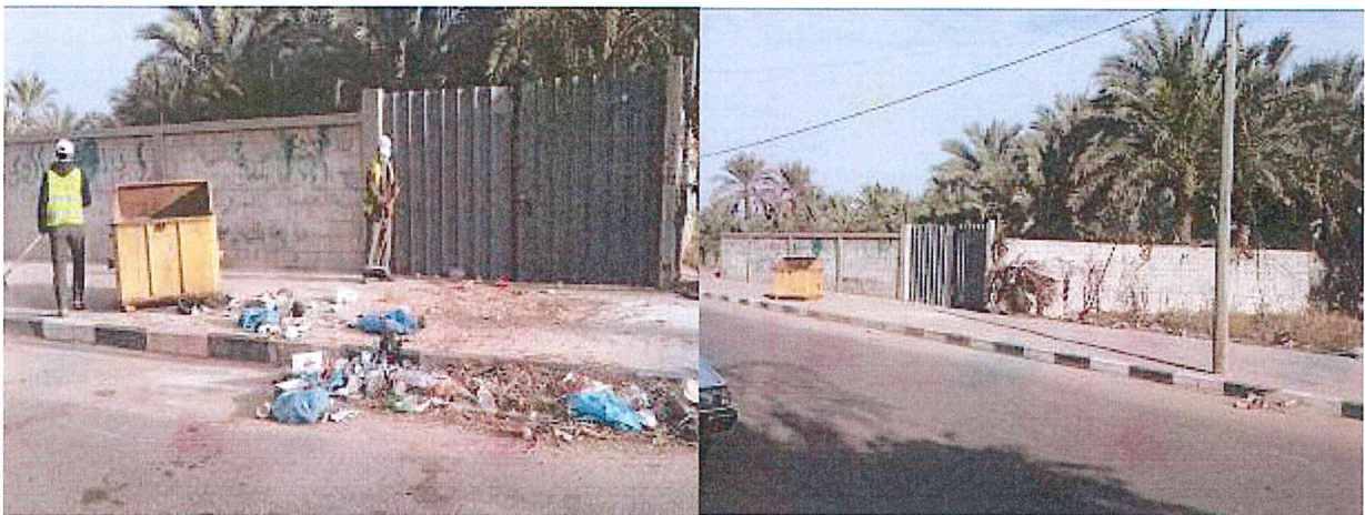
Construction debris & sand cleaning activity
