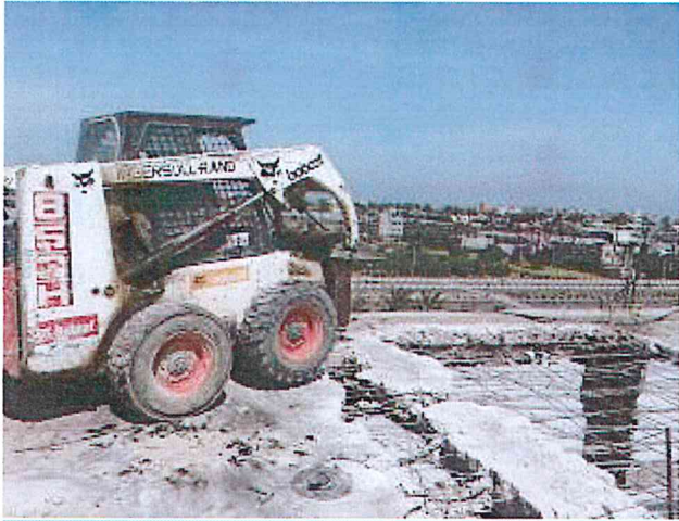
Rubble Removal Activities
