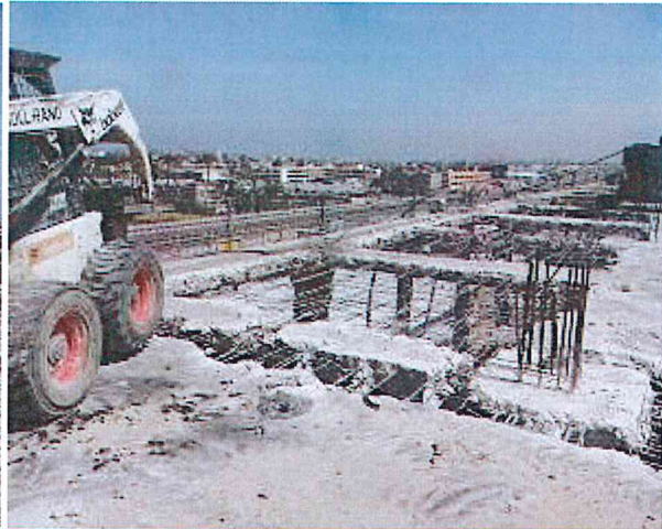
Rubble Removal Activities
